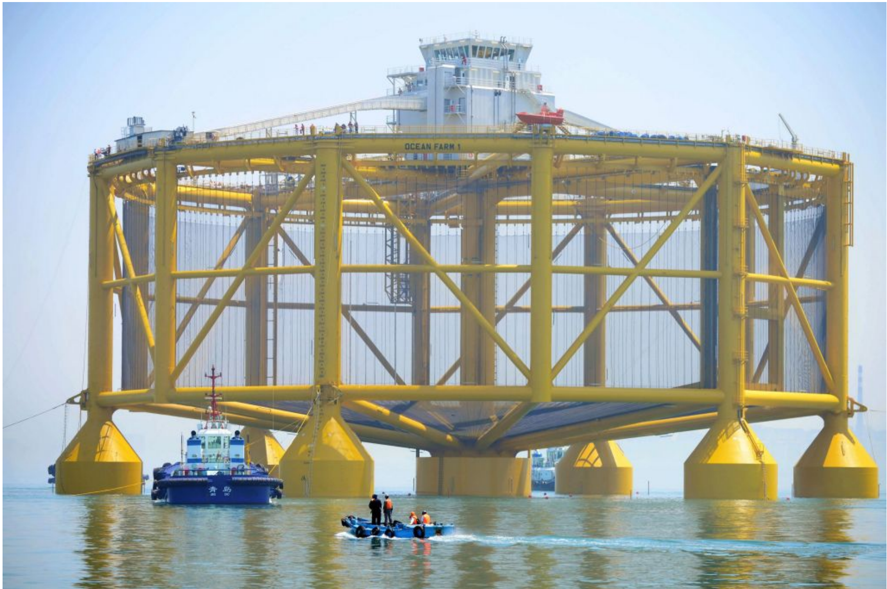
Figure 4: Ocean Farm 1 (picture) is already in operation. The Proposed concept of the largest yet to be built offshore aquaculture facility by SalMar ("Smart FishFarm") will dwarf Ocean Farm 1. Photo credit: Getty Images
